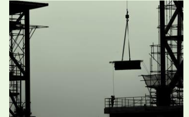
Concrete and construction
